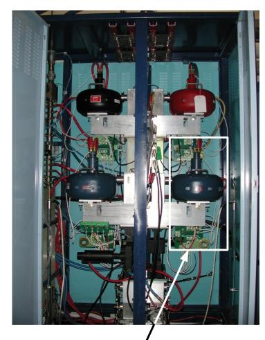
klystron and socket assembly
