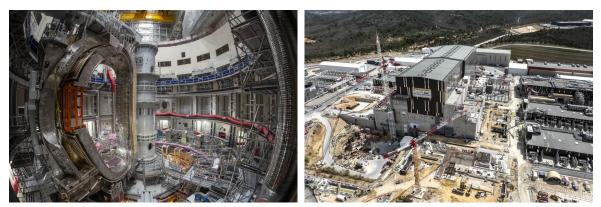
Figure 1.1. (Left, June 2022) The first vessel segment of the ITER tokamak, complete with two toroidal field coils, is in place in the tokamak pit; (Right, April 2022) aerial view of the ITER site
