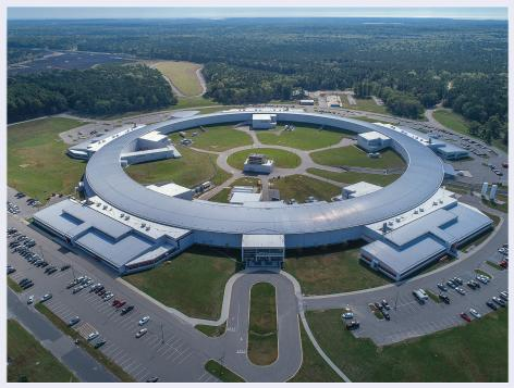
This aerial view illustrates the enormous scale of the recently upgraded Brookhaven National Laboratory's X-ray synchrotron. Electrons travelling near the speed of light in the circular magnetic storage ring are converted into X-rays for research use at dozens of individual experimental stations adjacent to the ring. (SOURCE: BROOKHAVEN NATIONAL LABORATORY)
